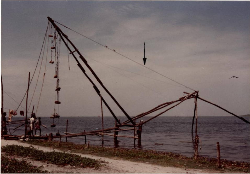
FIG. 4.7 'SAVAI'-THE LINES BETWEEN THE OUTER AND INNER CRANES.
