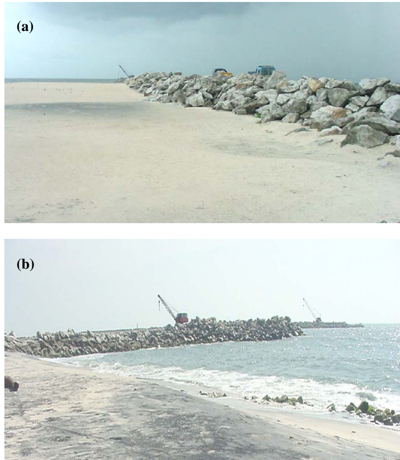
Fig. 5.10 Impact of breakwaters at Kayamkulam inlet: (a) accreted beach in the sector south of breakwater and (b) eroded beach north of the inlet
