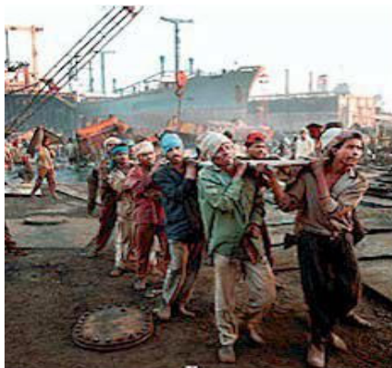
Fig.5.7 Manual Handling of Dismantled Hull Parts (Sibal 2001)
