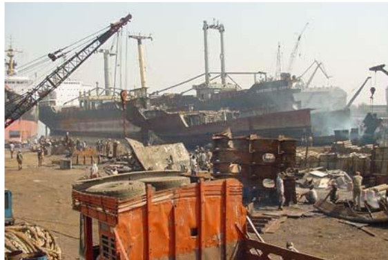
Fig 5.8 Buffering of Dismantled and Removed Items from the Vessel
