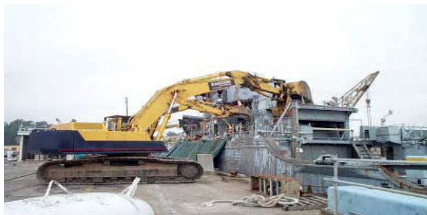
Fig. 2.3 Obsolete Ship Docked in Dry Dock for Dismantling (Sibal 2001)
