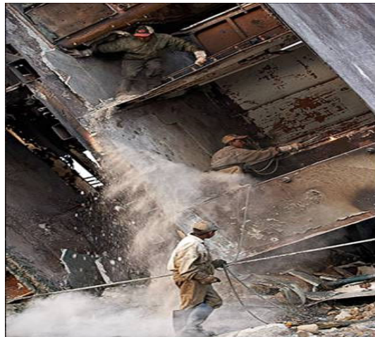
Fig 5.6 Oxy-Acetylene Cutting of Hull Parts (GMB)
